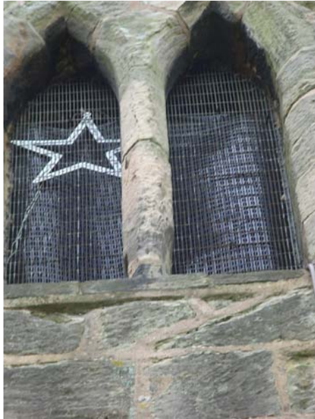
9.12 Eroded stone at bottom of mullion
