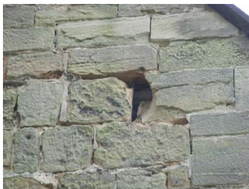
7.10 Hole in masonry near apex
