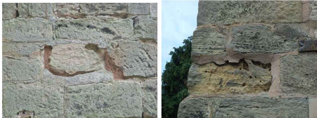
7.10 Damage by masonry bees
