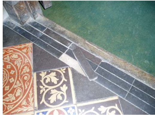
16.11 Loose tile slips by step down to vestry
