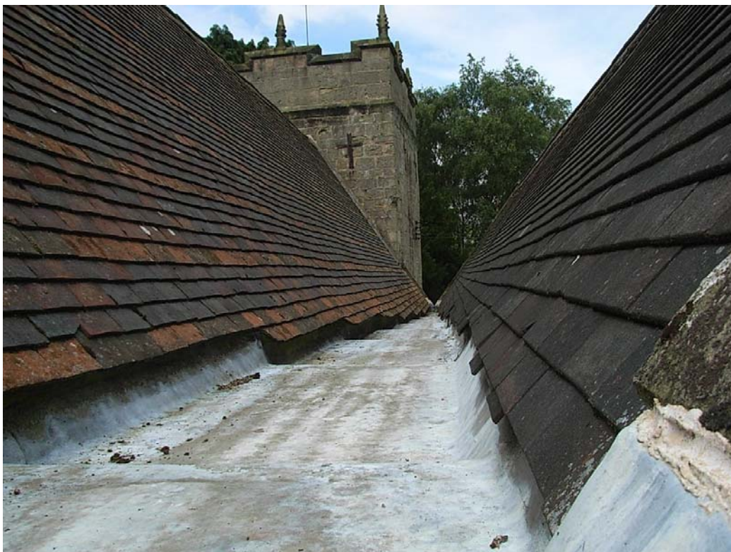
3.9 Slipped tiles on valley gutter
