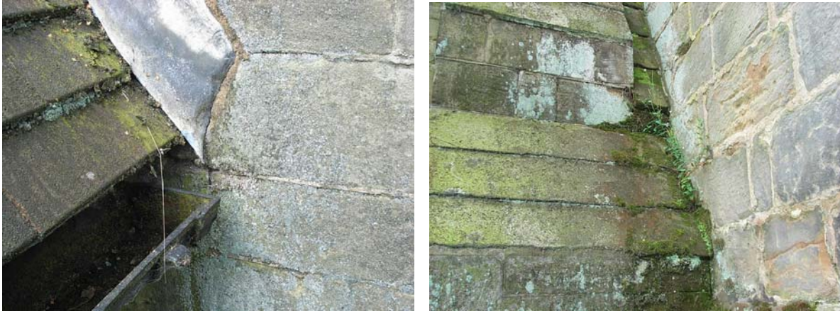
3.10 Water missing the gutter
