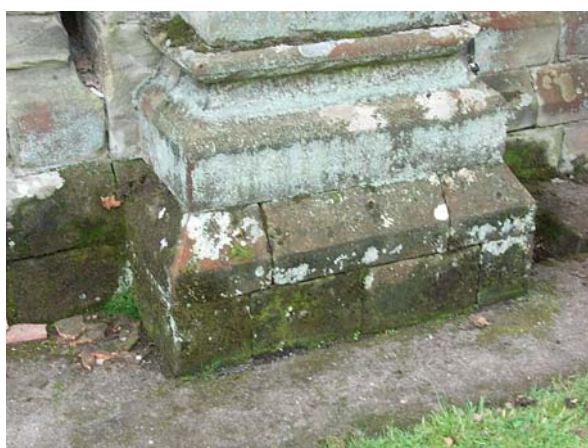
7.8 Buttress showing open joints
