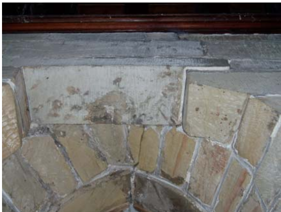
Crack above window in vestry
