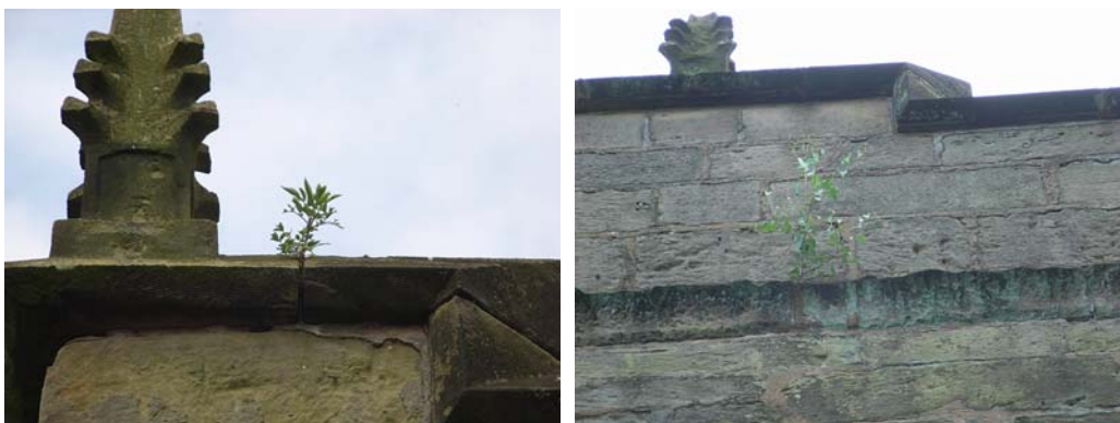
6.2 Vegetation growing in mortar joints
