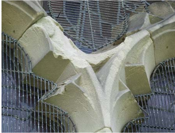
9.4 Eroded 'Y' section of tracery
