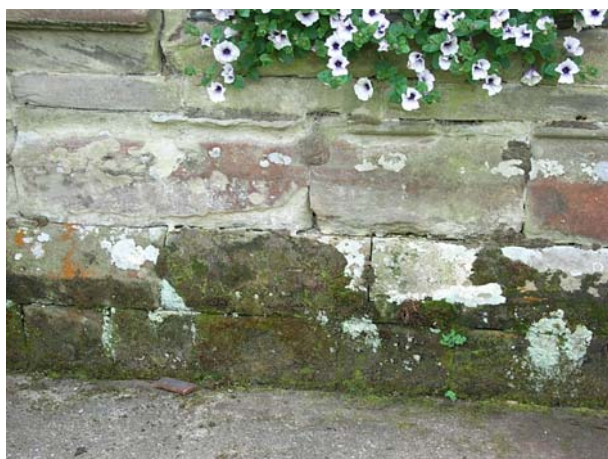
7.13 Open joints in plinth
