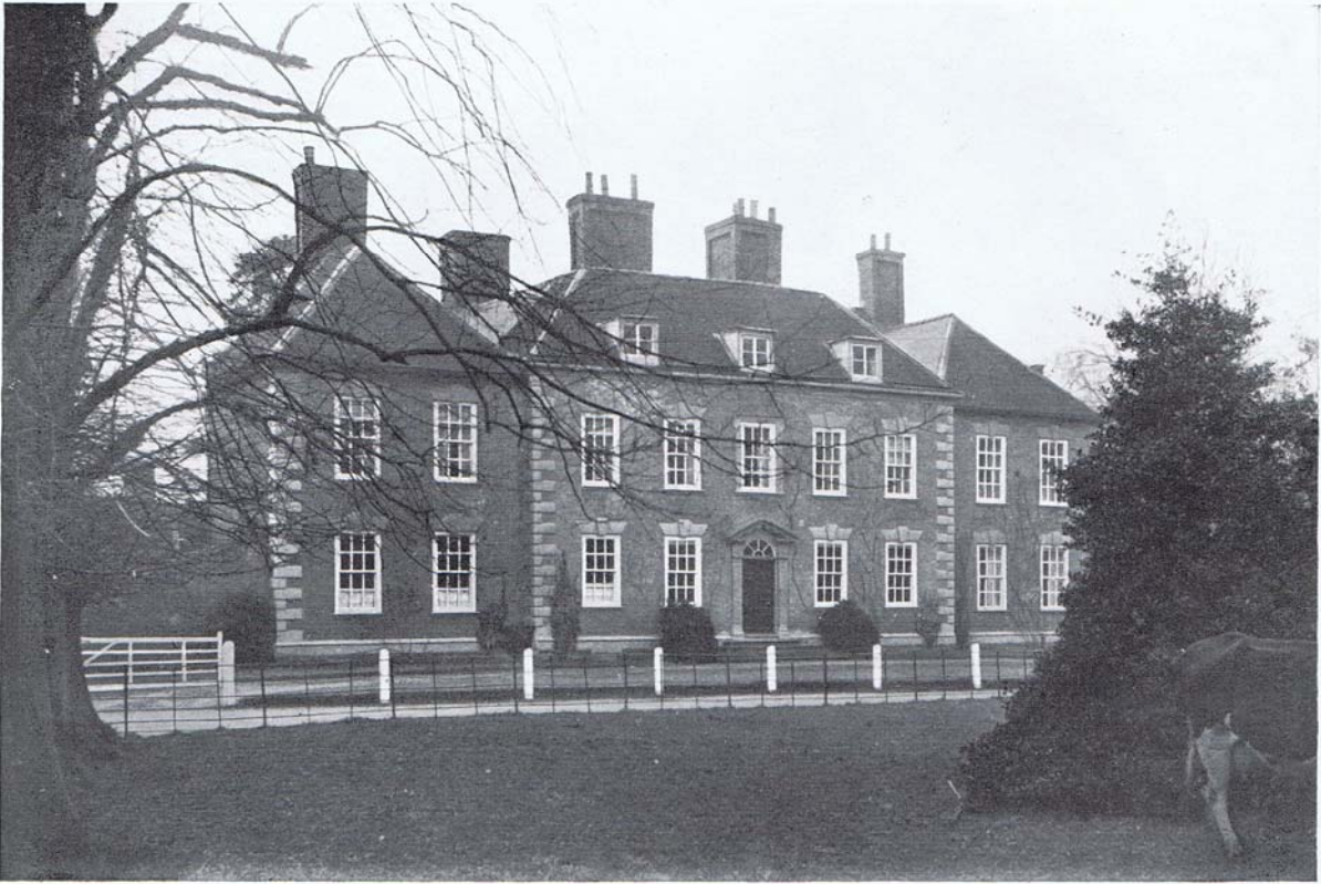
COLTON HOUSE. North Front. (Lot 11).
