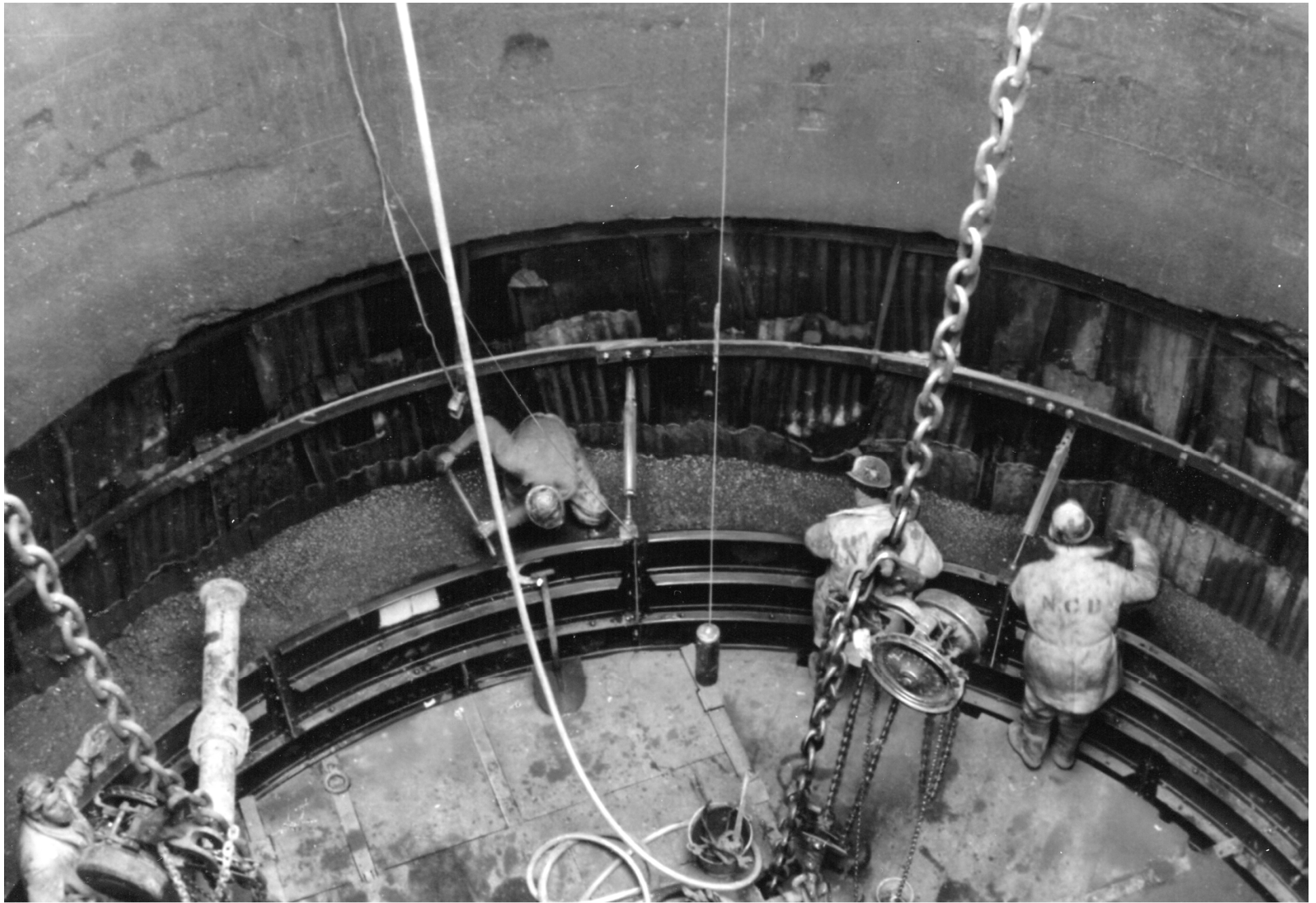
Constructing the concrete shaft wall.
