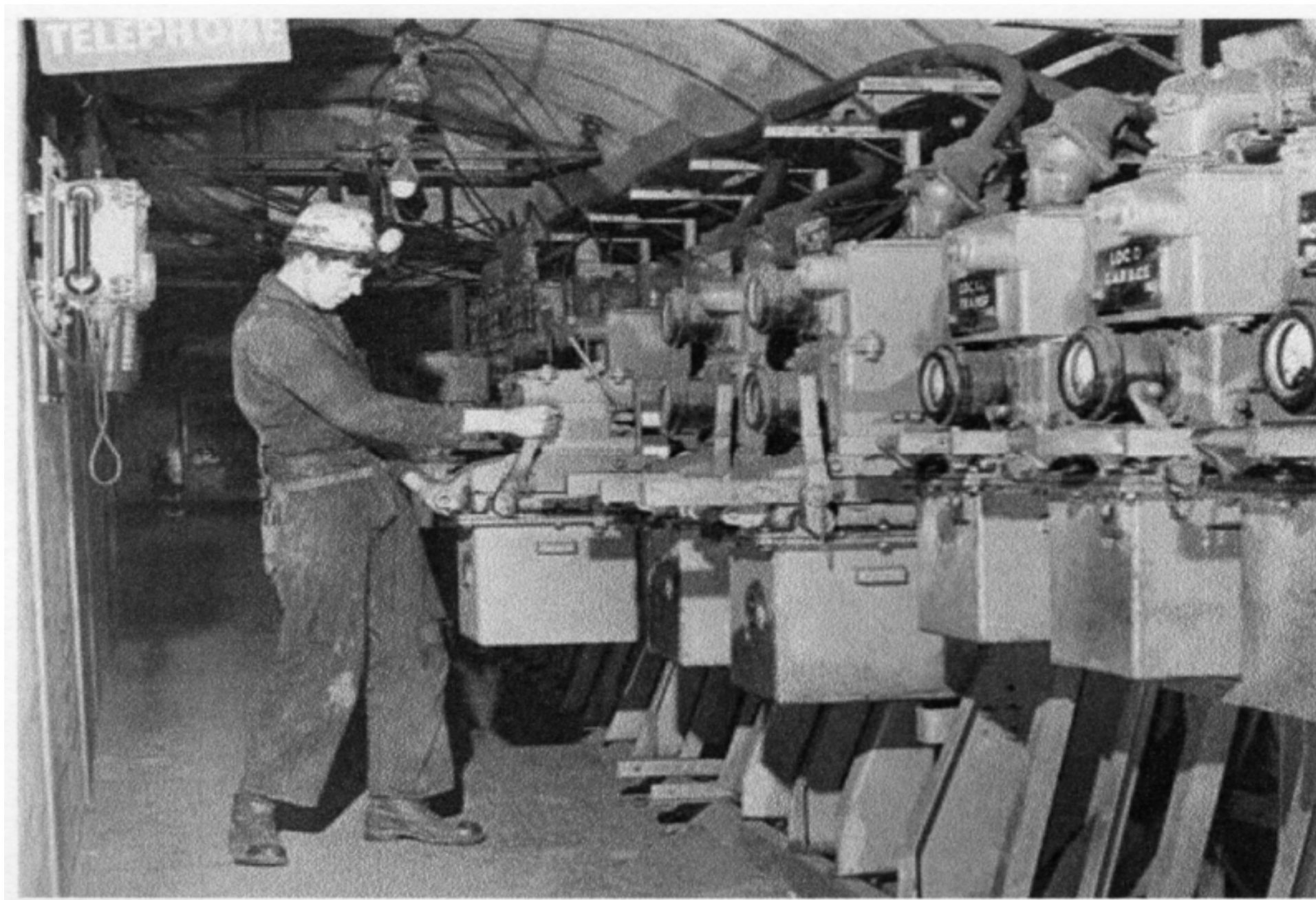
Underground 3,300 volt distribution sub-station c1965
