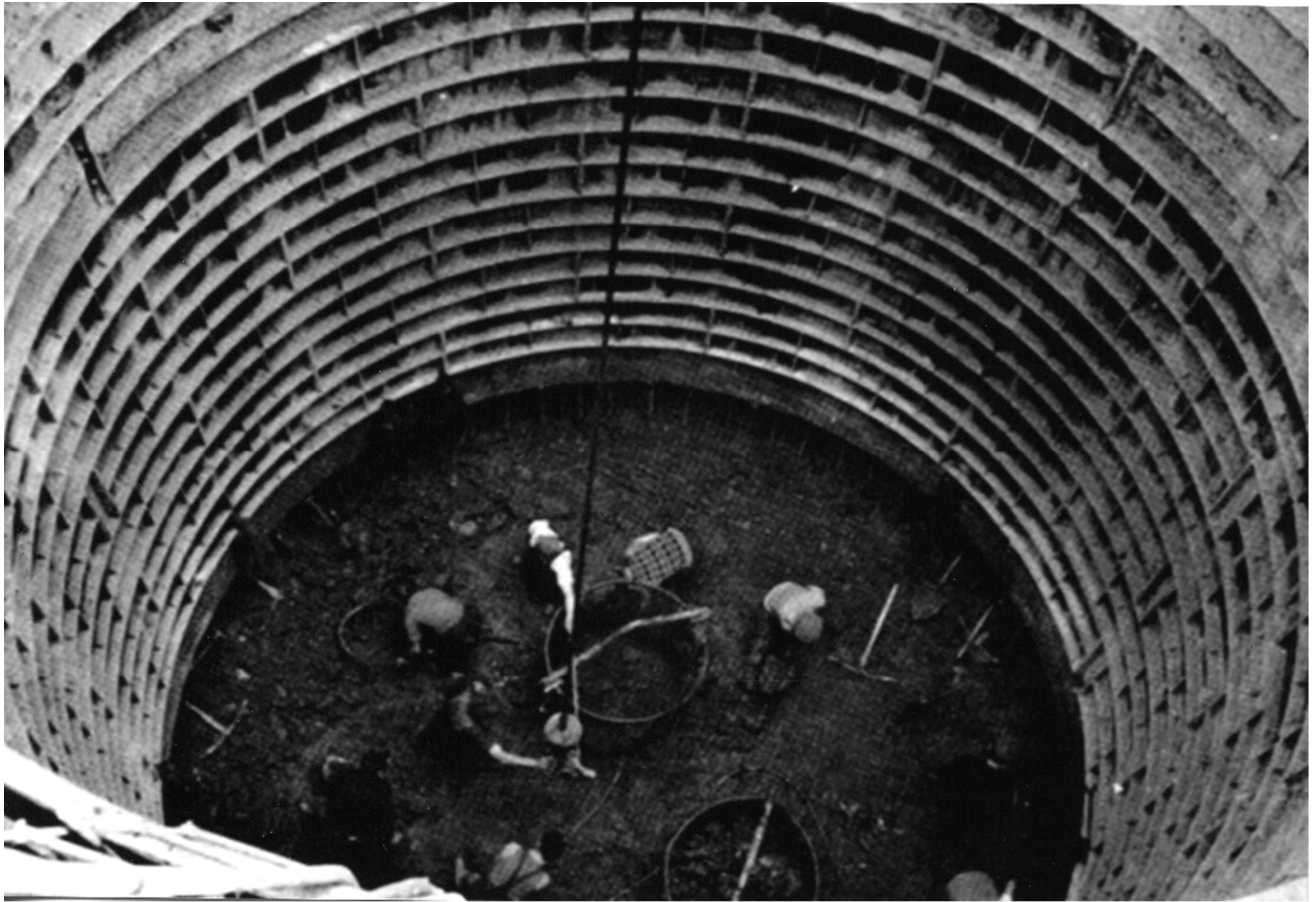
Shaft sinking in operation.
