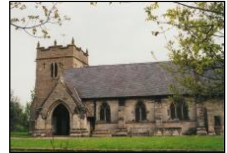
St Mary's South Entrance
