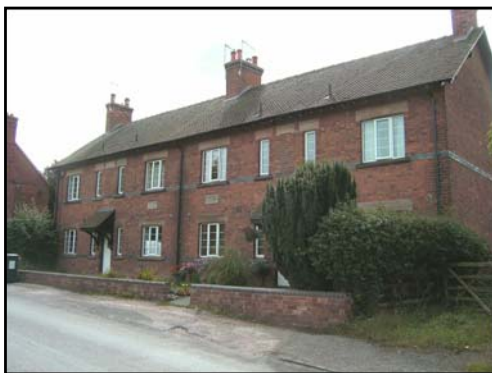
Oldham Cottages Refurbished in 2004
