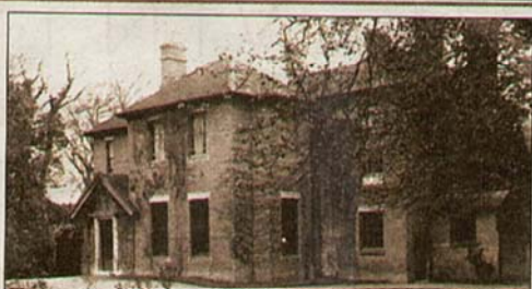
The Old Rectory was the oldest building in the village
